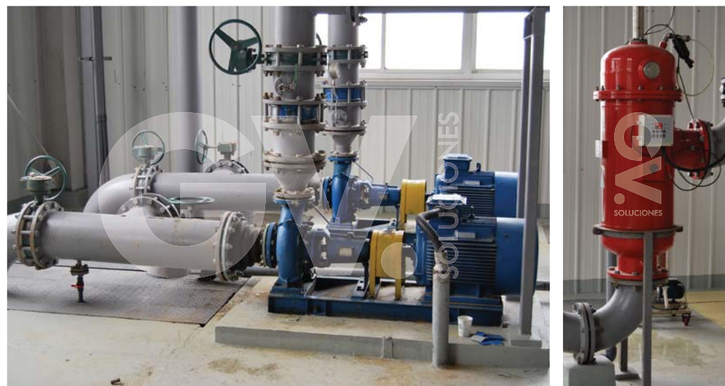
Membranas, bombas y filtro de planta potabilizadora. Membranes, pumps and filter of a drinking water treatment plant.
